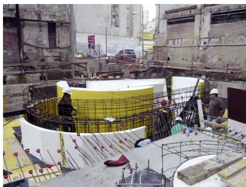
FROM THE STREET AND ENTRANCE LEVEL A SPIRAL STAIRCASE WAS INSTALLED LEADING TO A LOWER LEVEL MEANT FOR PUBLIC AREAS. A PARKING GARAGE OCCUPIES AN EVEN LOWER LEVEL.
